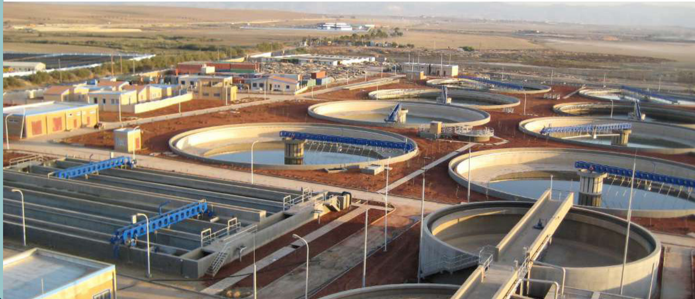
Building of a new waste water treatment plant of 270,000 m 3 /day. Oran, Algeria.
