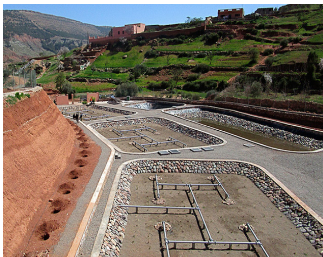
The project of waste water treatment in Asselda (Morocco) provides clean water to inhabitants and orchards.
