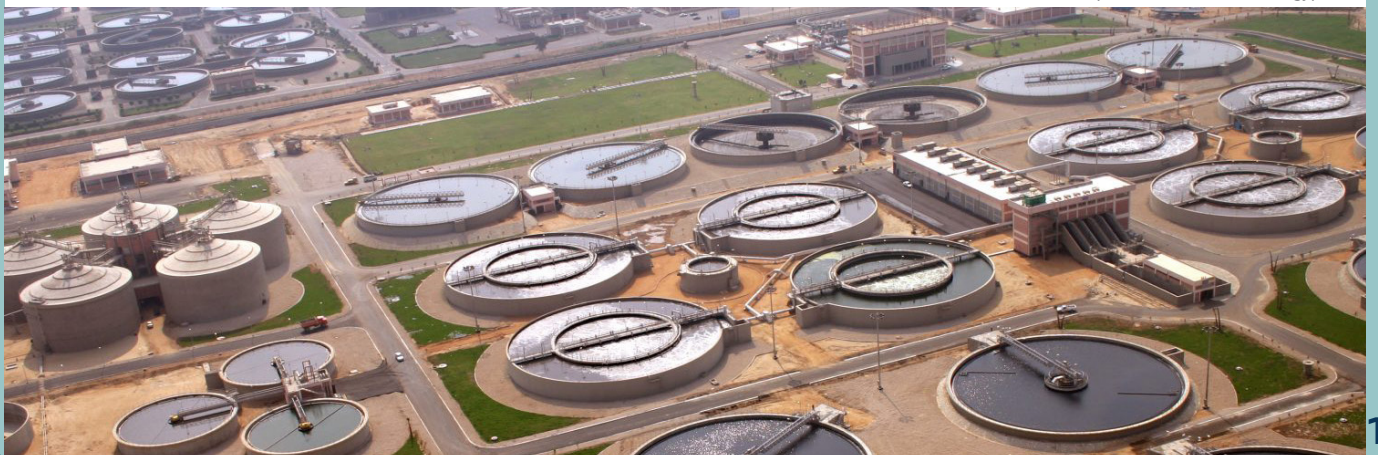
Waste water treatment plant of Gabal el-Asfar in Egypt.
